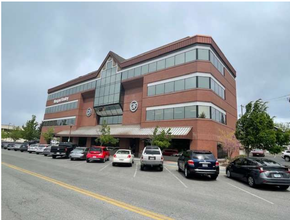
The Great Floors building conforms to Downtown Design Guidelines for material, color, and details.
